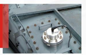
Qualitrol's drain valve sensor can be easily and rapidly retrofitted to the existing transformer oil drain / filter valve.
